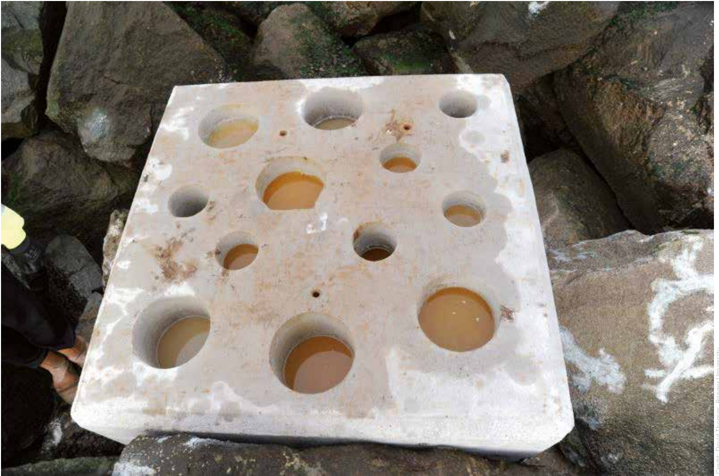
Figure 4.1 Bioblocks are habitat enhancement unit that create artificial pits and rock pools to provide habitat for native species.
