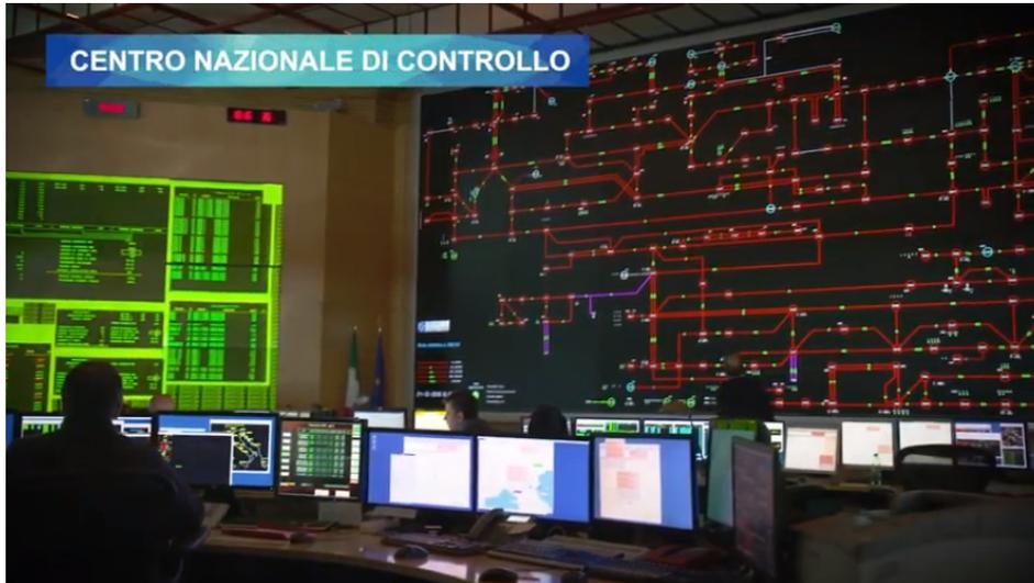
SCADA/EMS (Supervisory Control and Data Acquisition/Energy Management System)
